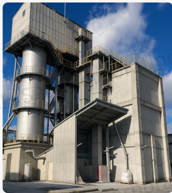
04. Coke-Fired Lime Kiln
