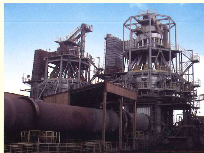
鉄鋼業用石灰石焼成 500ton/day、2002年2003年建設 Calcination of limestones for the iron and steel industry, 500 tons of product per day each, constructed in 2002 and 2003
