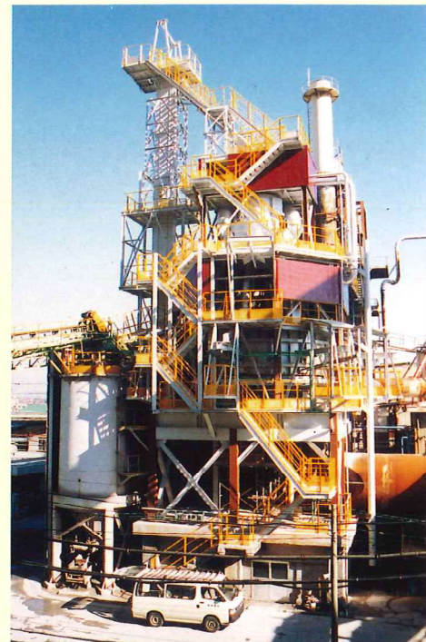
石灰石の化学工業用高品質焼成 220ton/day、1998年建設 High-quality calcination of limestone for the chemical industry, 220 tons of product per day, constructed in 1998
