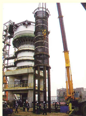
内筒上架・挿入 HANGING UP AND POSITIONING OF INSIDE COLUMN
