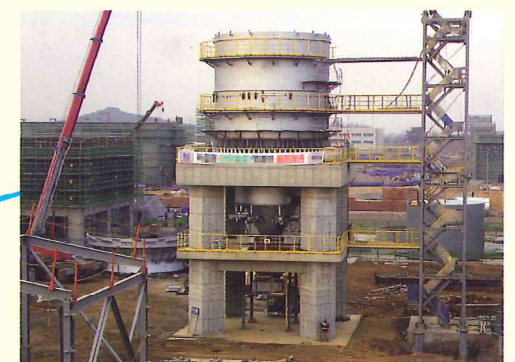
第二段鉄皮据付 INSTALLATION, SHELL OF SECOND LEVEL
