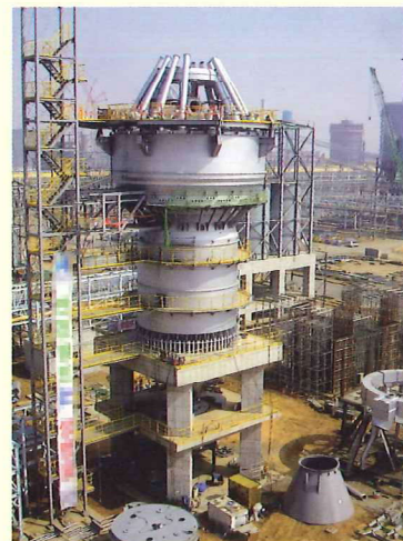
原石パイプ据付 INSTALLATION OF CHARGING PIPES
