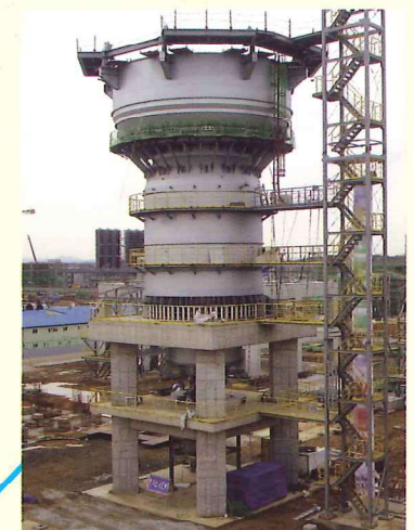
予熱帯鉄皮据付 INSTALLATION, SHELL OF PRE- HEATING ZONE
